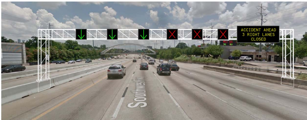
ES Figure 2. An Example of a Proposed Sign Bridge for the Corridor with DMS and LCS
